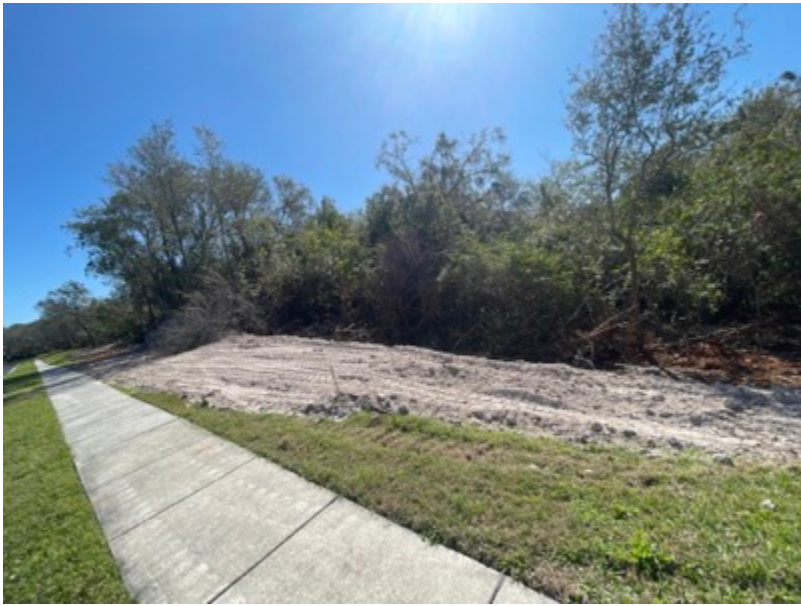
Facet View Common Area Property Manager Work being completed on common area along facet View. Work not being completed by yellowstone
